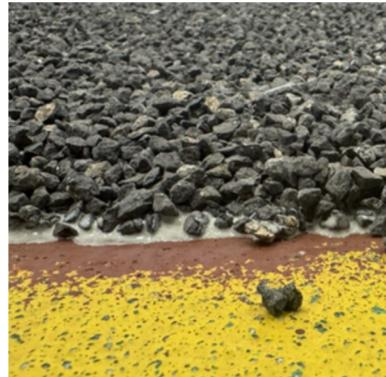
Loose and unbound aggregate must be removed once the coating has cured sufficiently to withstand foot traffic.
